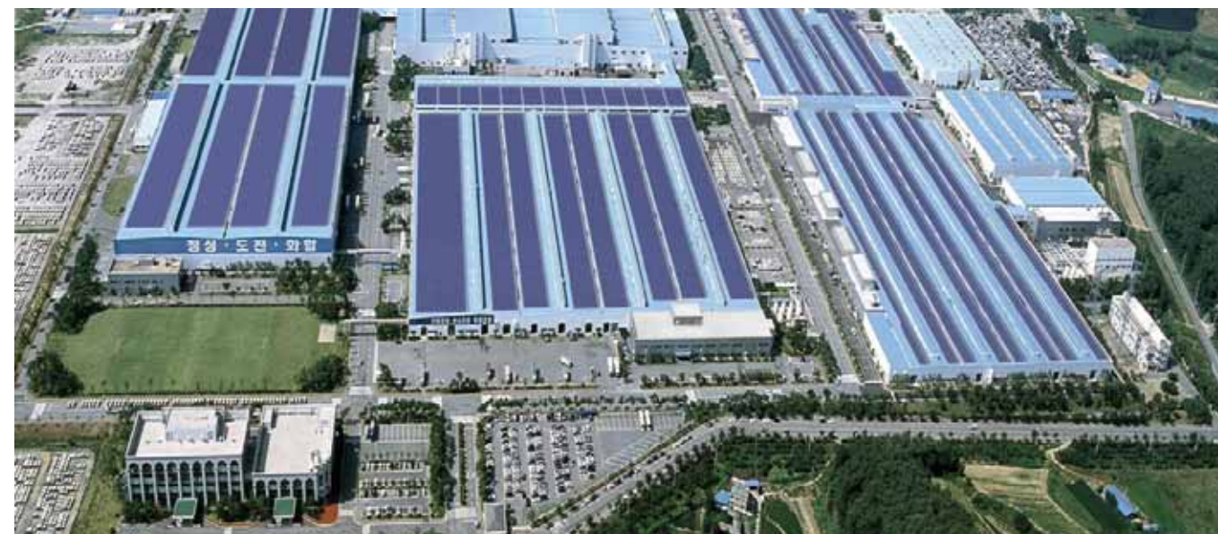
Hyundai has partnered with a local power company to install solar panels on the roof of the Asan plant for clean GHG-free electricity generation. It is the second largest rooftop solar facility in the world.
