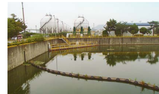
Pollution Prevention Facilities - Monitoring Pond
