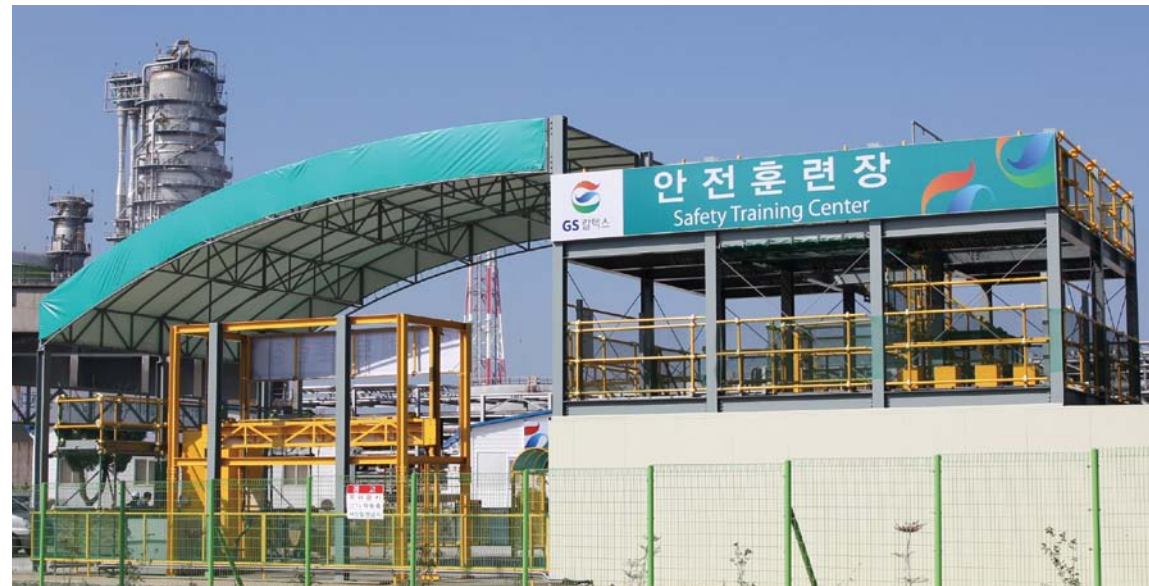
GS Caltex Safety Training Center
