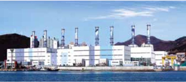
Busan Combined Cycle Power Site ● Address: Gamcheonhang-ro 7, Saha-gu, Busan Metropolitan City ● Fuel: LNG ● Installed Capacity: 1,800MW (G/T 150×8 units, S/T 150 × 4 units)
