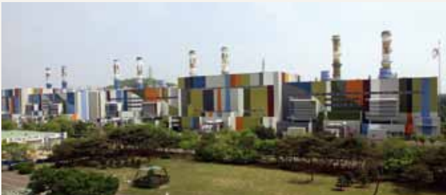
Shinincheon Combined Cycle Power Site ● Address: Jangdo-ro 57, Seo-gu, Incheon Metropolitan City ● Fuel: LNG ● Installed Capacity: 1,800MW (G/T 150×8 units, S/T 150×4 units)
