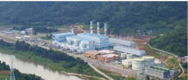
Yeongwol Combined Cycle Power Plant ● Address: Joongang-ro 411, Yeongwol-eup, Yeongwol-gun, Gangwon-do ● Fuel: LNG ● Installed Capacity: 848MW (GT 183×3 units, ST 299×1 unit)
