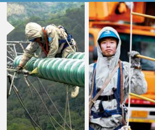
ZHENG Ruidong changing the insulator on 500kV high voltage transmission lines.
