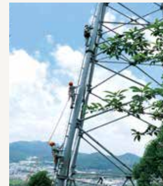
On-load Operation of 500kV Compact Transmission Lines
