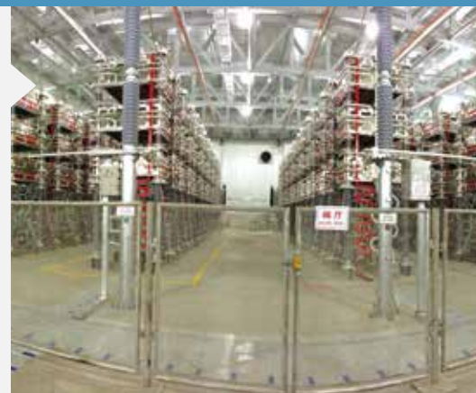
Multi-End Flexible DC Transmission System Converter Valve ▲
