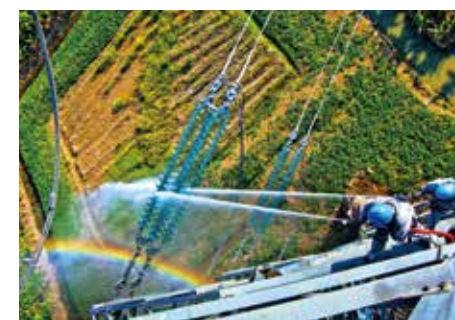
Washing power equipment in the air ▲
