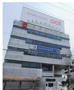
kt's Banghak Office Powered by Geothermal Energy
