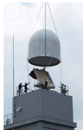
Weather radar being constructed
