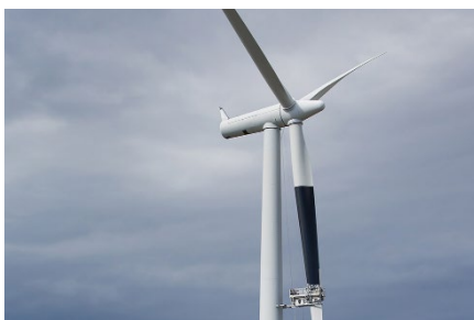
In 2013, trials started at Smøla wind farm to make the wind turbines more visible to birds through use of lights or contrast paint. The goal is to reduce the risk of bird collisions. The trials are a collaboration with Statoil, Vattenfall, Trønder EnergiKraft, NVE, the Research Council of Norway and Energy Norway, and are carried out by the Norwegian Institute for Nature Research. Photo: Espen Lie Dahl
