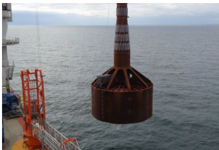
The Bucket Foundation is lowered into the sea at Doggerbank
