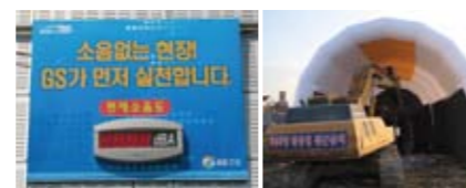
On-site noise level measuring board Air soundproof wall
