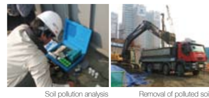
Soil pollution analysis Removal of polluted soil
