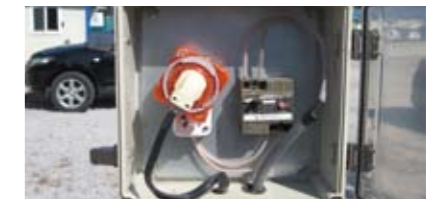
Nangang Dam Upstream Sewer site
