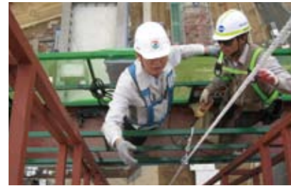
Checking the gondola for installing outside structure
