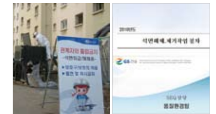
Asbestos abatement work Asbestos Abatement Manual
