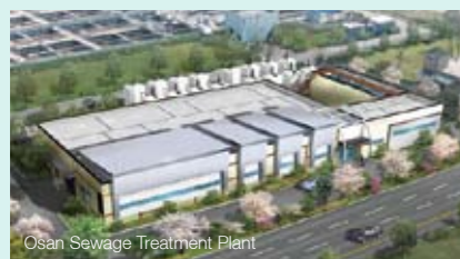
Osan Sewage Treatment Plant
