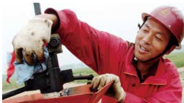
A worker from Sinopec Zhongyuan Oilfield is maintaining an oil well. There are environment-friendly toilets and dustbins for different garbage for all drilling teams with no discharge of waste water and castoff. On all construction sites, ecological protection standards were met and 100% of pollutants recovered
