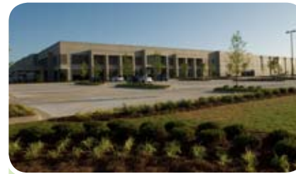
Social Circle, Ga., distribution center
