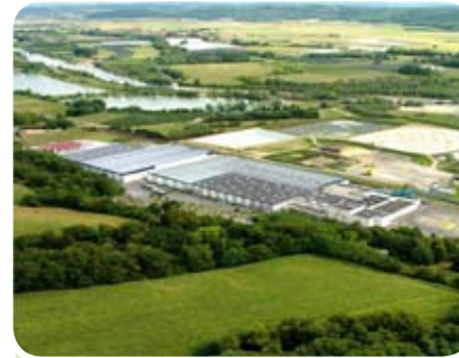
Seretram facility in Labatut, France
