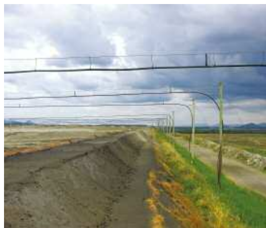
Dust suppression measures, in the form of overhead irrigation, on tailings facility three, four and five at our Marikana operations.
