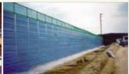
Measures to Reduce Air Pollution at Construction Sites Operate vehicle-washing facilities Temporary dustproof fences
