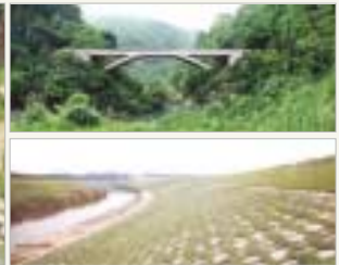
Measures to Manage Water Channels & Water Supply Left: Move waterways, retaining their natural form Right: Acquire sites for the natural flow of waterways: set up environmentally friendly bank-protection blocks
