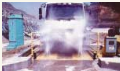
Measures to Reduce Air Pollution at Construction Sites Operate vehicle-washing facilities Temporary dustproof fences
