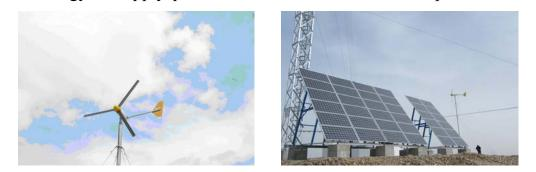
major supply in the daytime and wind will provide power in rainy days and evenings. Currently 76 base stations with wind and PV hybrid technology have been built up, which are expected to save 1.976 yuan in maintenance each year.
