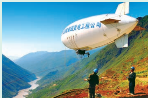
Airship Stretching to Reduce Impact on Vegetation
