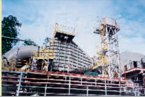
Bag filter for atmospheric emission control.
