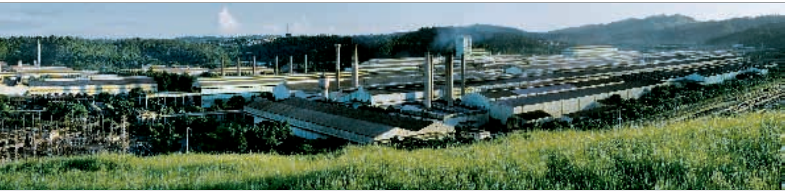
View of Intendente Câmara Steel Mill in Ipatinga – MG.
