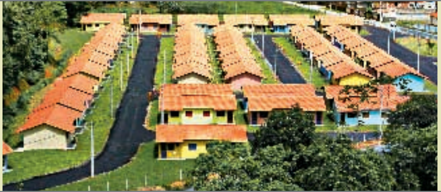
Houses at Areal Condominium in Angra dos Reis (RJ) built with Usiteto technology.
