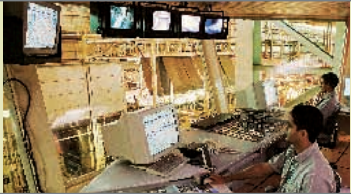
Rolling Mill Control Room – Intendente Câmara Steel Mill.
