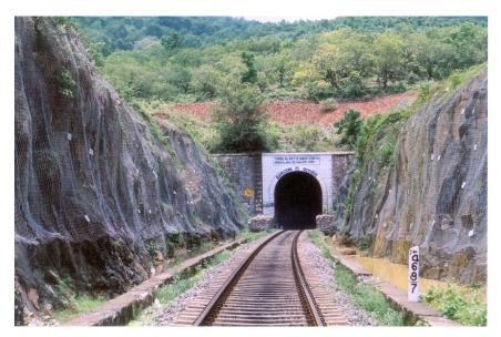
Boulder Netting and Geo-safety works have been carried out on a large scale throughout Konkan Railway route to strengthen the cuttings and to protect the environment.
