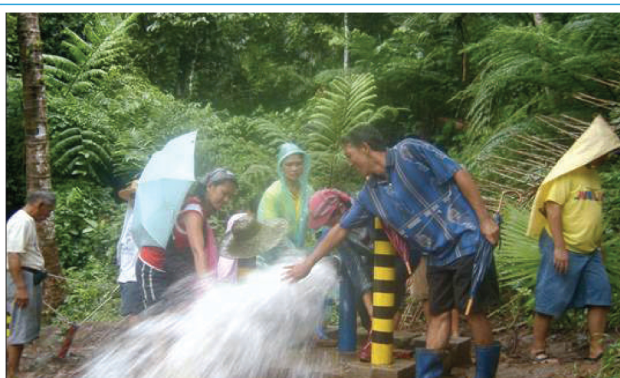
Water Supply project in Cavinti, Laguna
