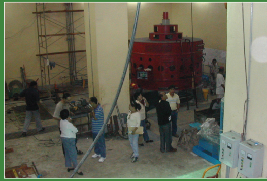
Sevilla mini-hydro power plant, in Bohol, showing one of the "Two units (2 x 1 250 KW) Vertical Flexible Kaplan turbines" connected to a two units (2x 1 250 KW) 6600 Volts, 60Hz Synchronous Generators and associated controls.
