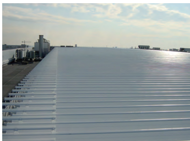
Roof of plant building after applying insulation paint
