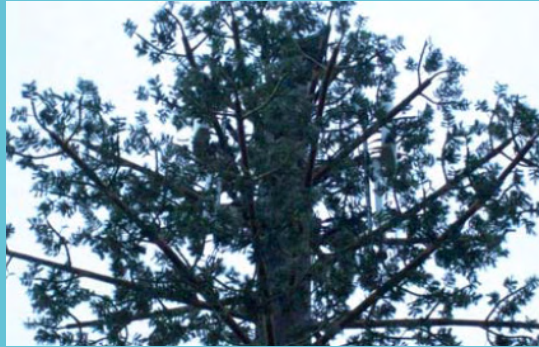
An example of a mobile communications tower camouflaged under a structure that simulates vegetation
