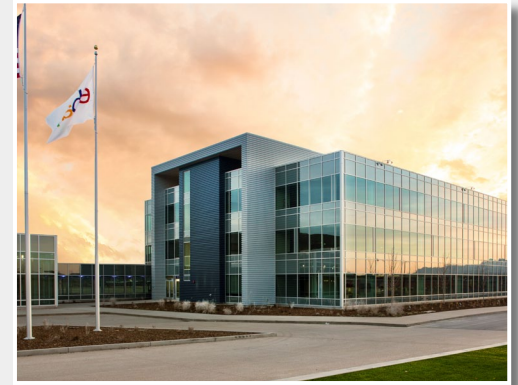
Our third LEED Gold-certified building in Draper, Utah was awarded a Business Sustainability Award from Utah Business Magazine in November 2013. Photo courtesy of Scot Zimmerman.
