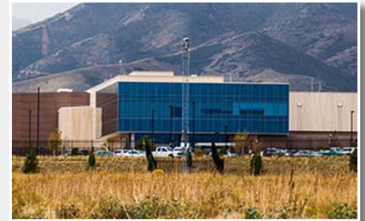
Our newest data center opened in September 2013 in Salt Lake City, UT.
