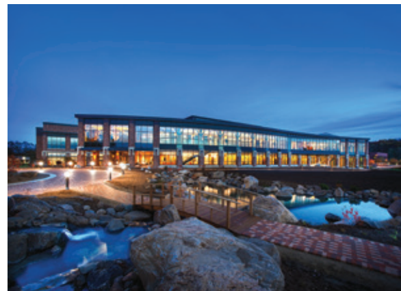
The Feynman Center, above, added 260,000 ft 2 to Promega's global building footprint.
