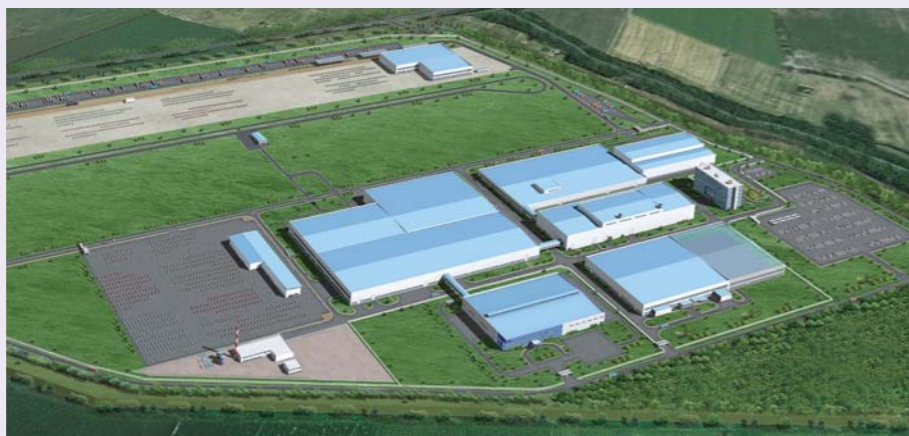
Full View of Czech Plant
