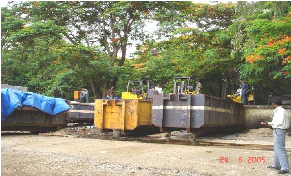
Photo: A view of the Common Intermediate Hazardous Waste Transfer Facility, where hazardous waste is transferred from our dumper trucks directly into the custom built containers of CHWTSDF– Taloja.
