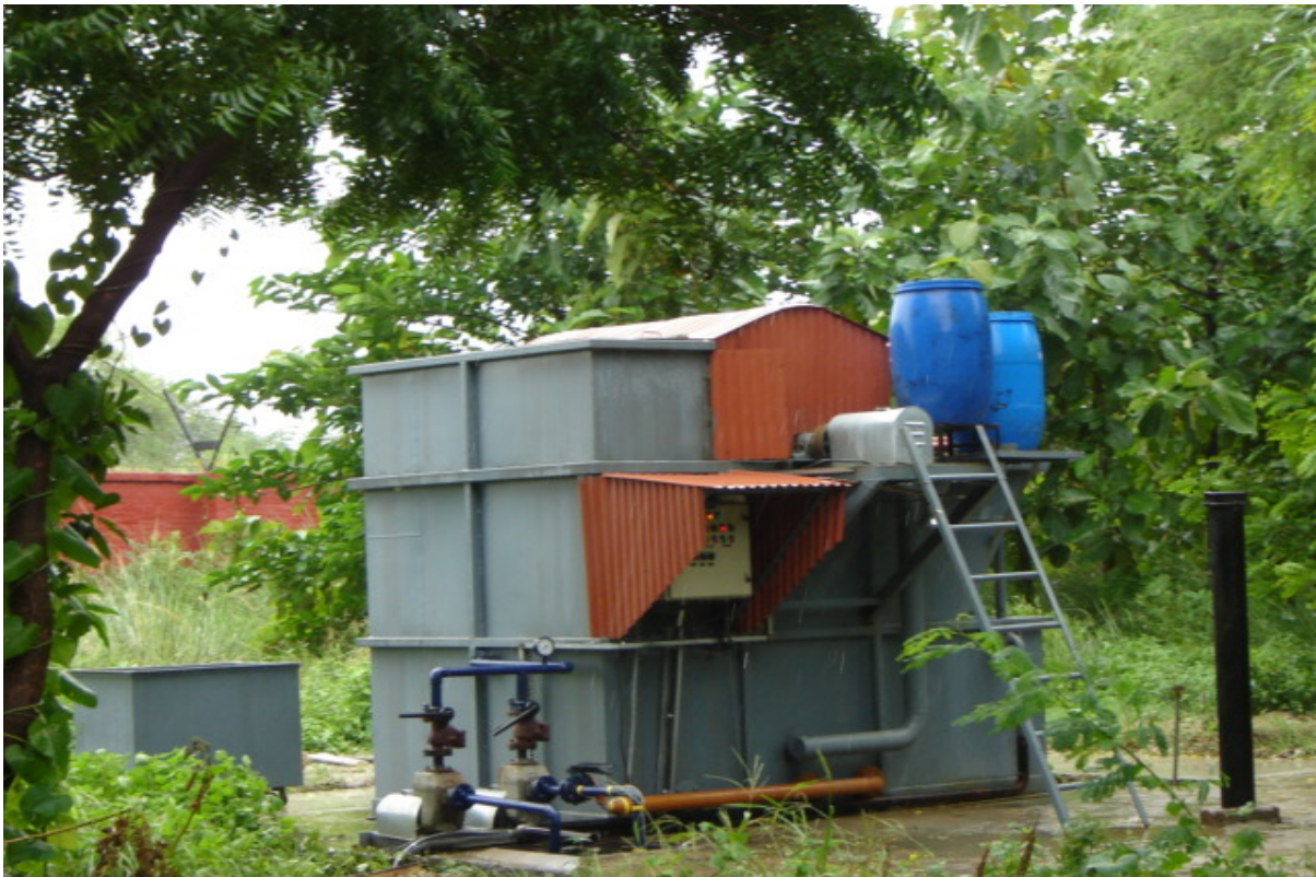
Fig.: Sewage Treatment Plant Installation at Lucknow Plant
