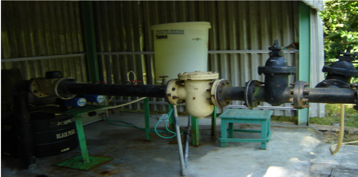
Fig.: Improvisation in Water purification System by substituting Bleaching Powder with Sodium Chloride
