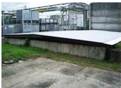
Roof covering treated water storage pool
