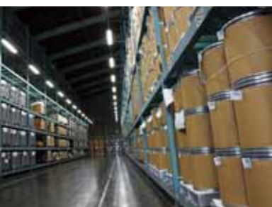
Osaka Plant: Storage building for raw materials and packaging materials
