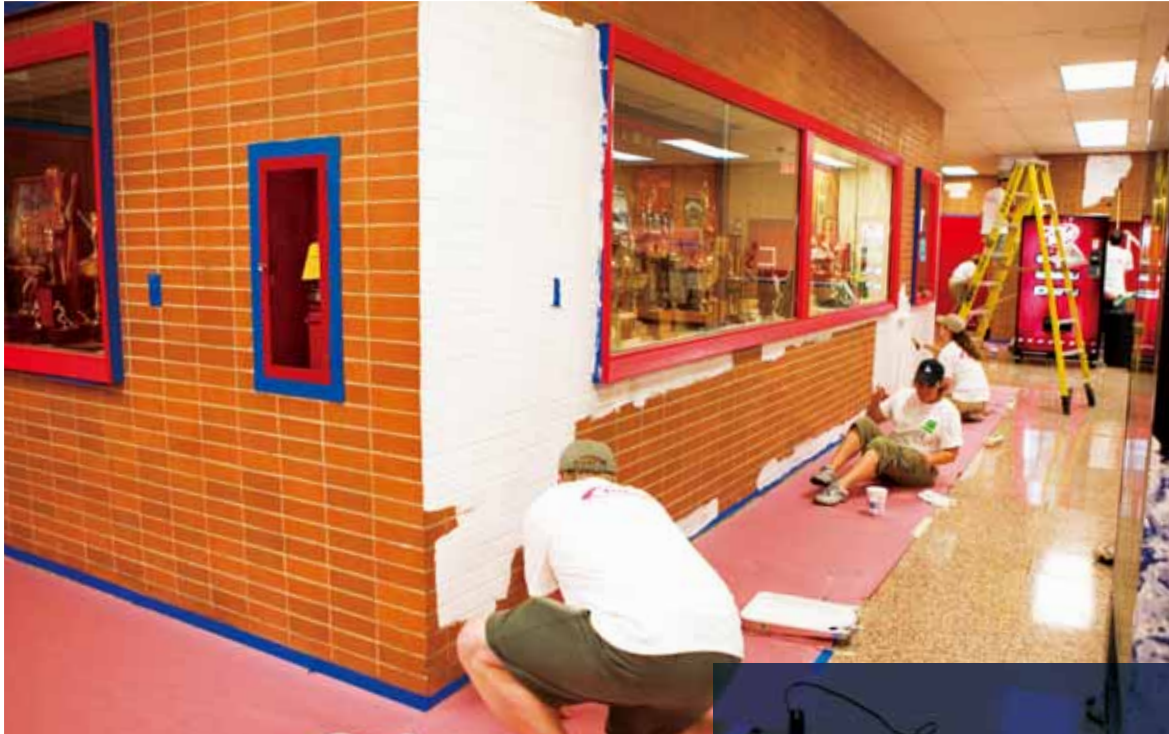
TPNA employees apply a new coat of paint to brighten up a wall
