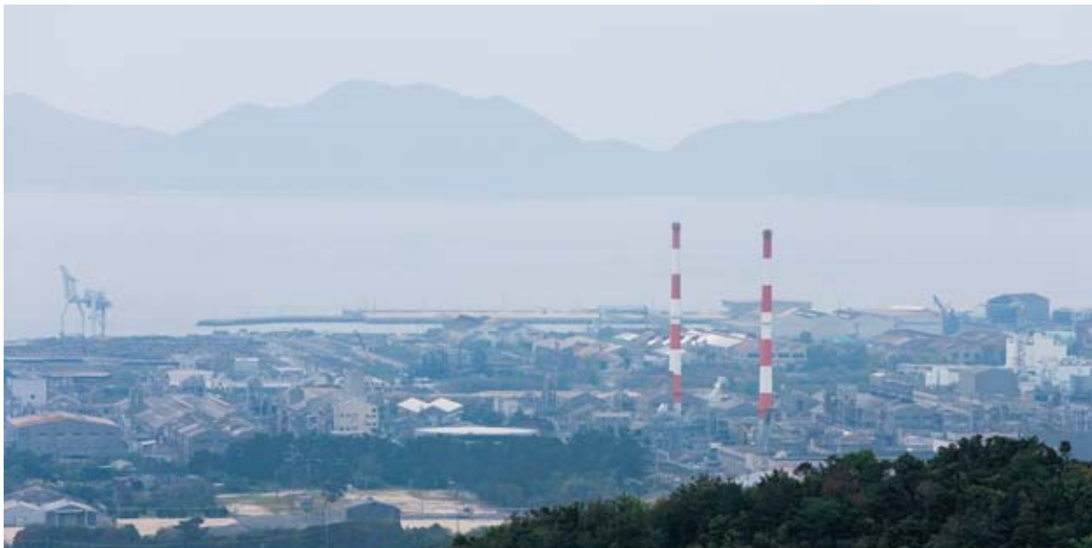
The Hikari Plant uses a sophisticated management system to protect water and air quality, ensuring harmony with the beautiful nature of the nearby Setonaikai National Park.
