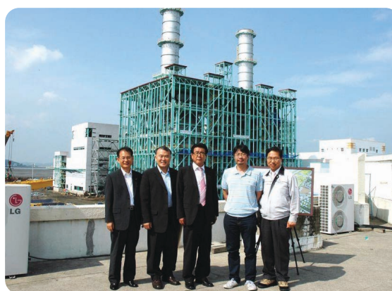
▲ Field Inspection by Non-standing Director (Gunsan CC Power Plant Construction Site / June 2009)
