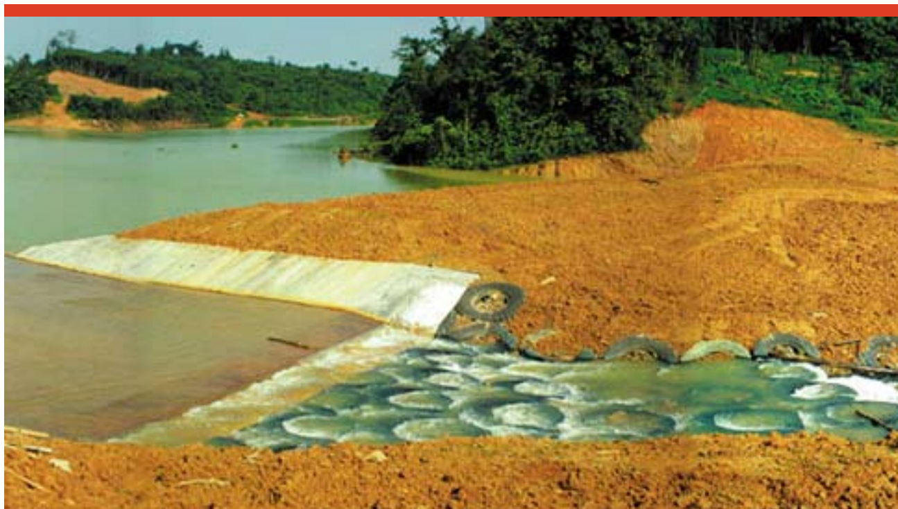
Graphic 37. Lower Melaso Pond with drop structure from used tires
