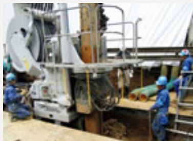
Extension work of the water-shielding wall
