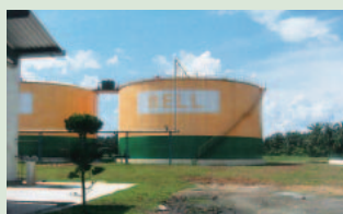
The anaerobic biogas digester, recovering methane from the effluent
