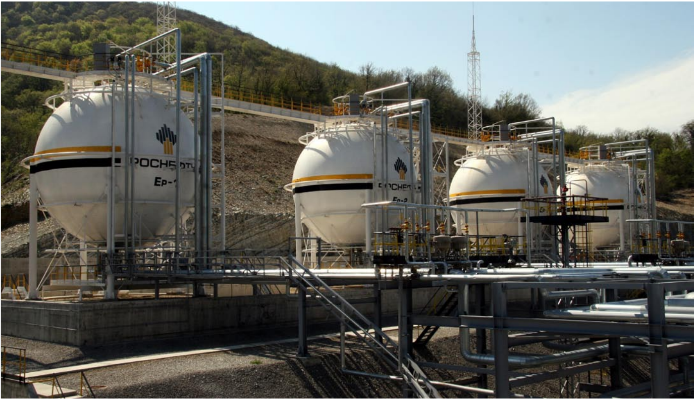
Liquefied gas reservoirs at Tuapse refinery
