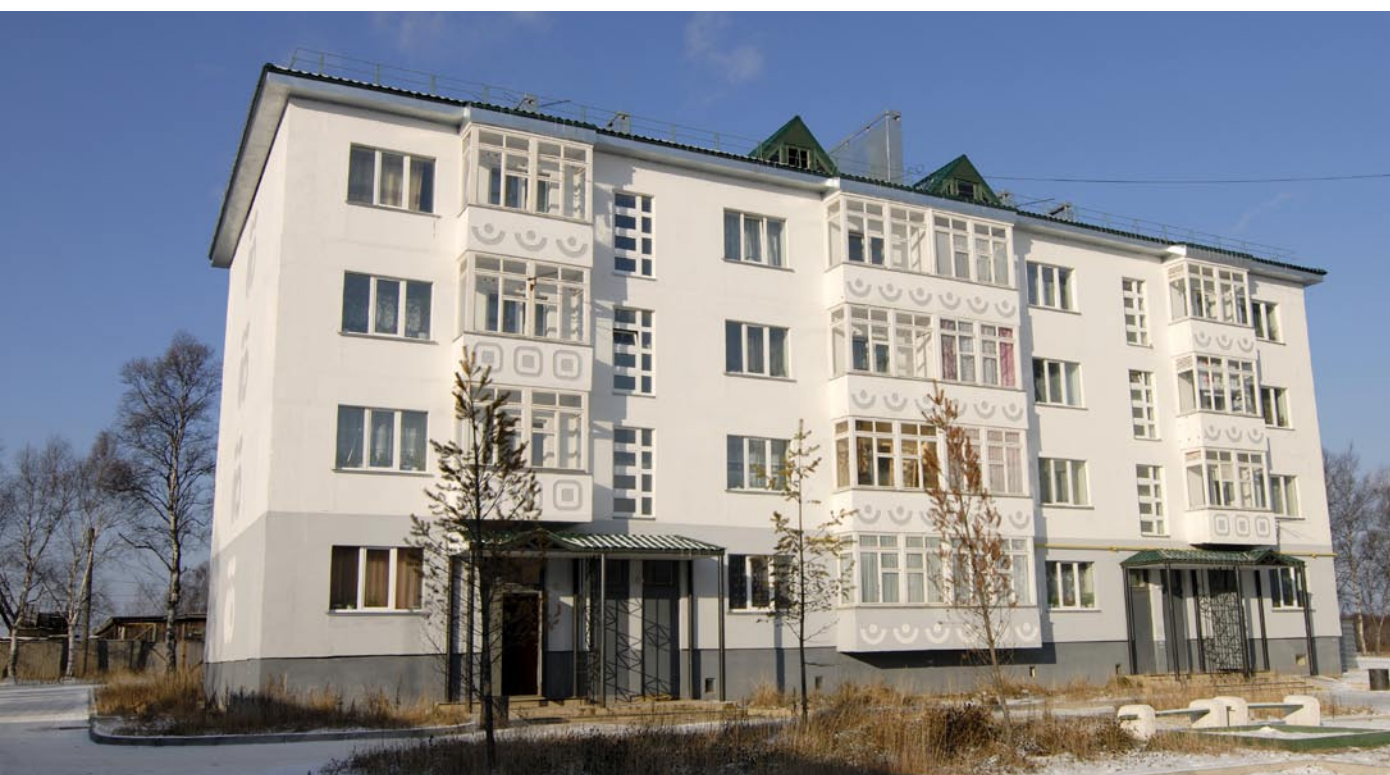
Residential house on Sakhalin, construction of which was financed by Rosneft
