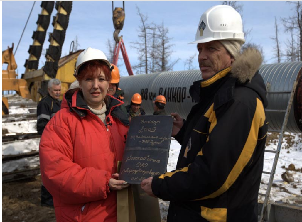
The symbolic final weld of Vankor-Purpe pipeline is complete
