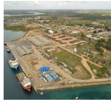
Supply base at Mtwara Port
