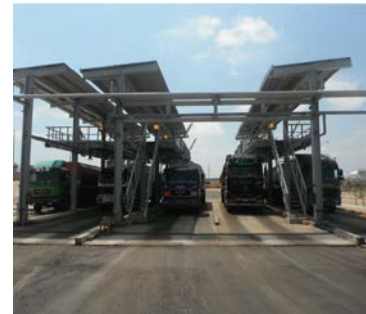
Trucks transporting water for treatment at our Egyptian operations
