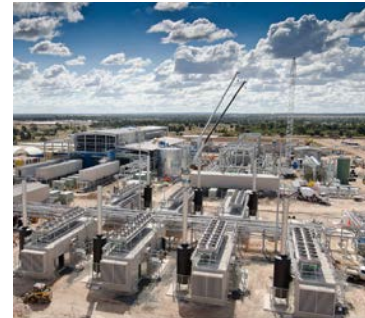
Kenya water treatment plant, Queensland
