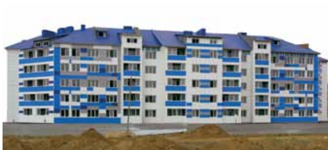
Kotelnikovo. Dormitory for 60 families
