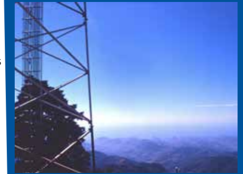
Hybrid battery solutions Hybrid battery solutions combine solar power, deep cycle batteries, turbines and fuel energy sources. By alternating between different power sources, hybrid batteries help us save significant amounts of fuel at off-grid sites.
