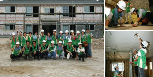
Volunteer activity - Building houses for the underprivileged
