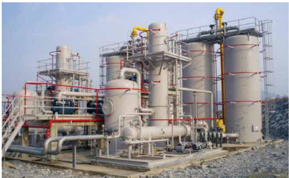
Installed oil vapor treatment system in Yeosu office
