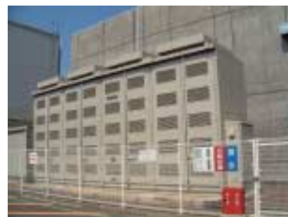
Figure 3: NAS Batteries Used to Store Nighttime Electricity
