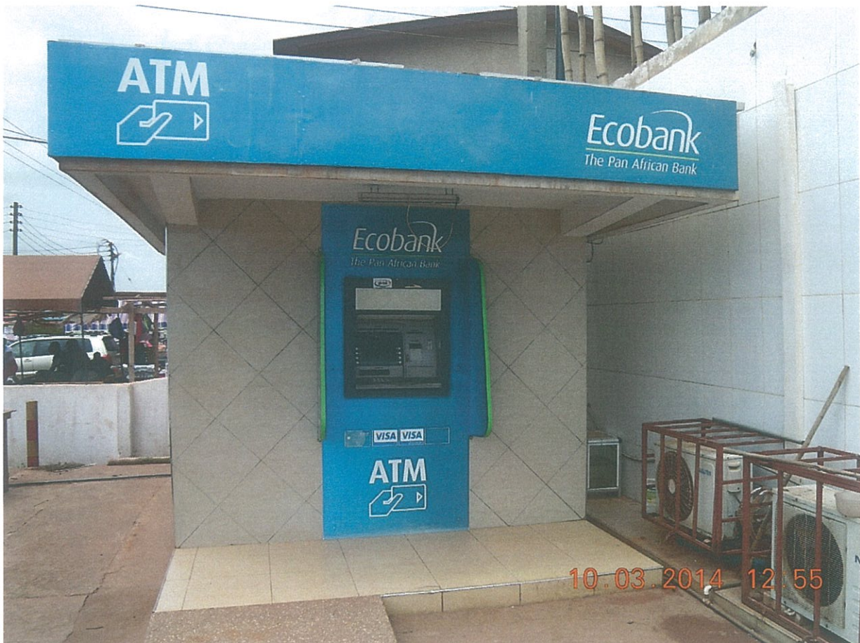
Figure 3: Solar powered ATM
