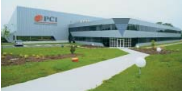
The Process Conception Ingénierie plant in Rennes (France)
