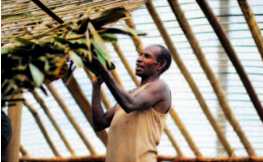
Building a new church, Gulesa, Hela Province.
