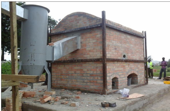
Plates 76 and 77: Shows GMC assisted incinerator under construction at the Fiaseman Senior High School, Tarkwa.
