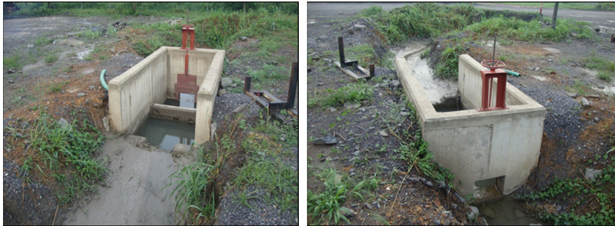
Plates 12 and 13: ingress and egress sections of the storm water drainage with pen stock valve
