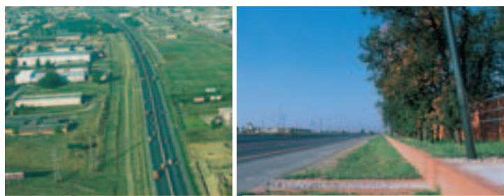
BEFORE/AFTER: A64 Toulouse to Muret, a successfully redesigned city entrance.
