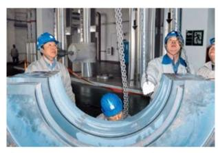
Efficiency improvement was carried out on cylinders of 47 units with installed capacity of 14,735MW and the heat consumption was reduced by 206 kilojoules/ kWh after the overhaul, equal to a drop of coal consumption for power supply by 8.36 g(standard coal)/kWh. As a result, the consumption for power supply of the rest units decreased by 2.273 g(standard coal)/kWh and 400 thousand tons of standard coal was saved in 2008.
