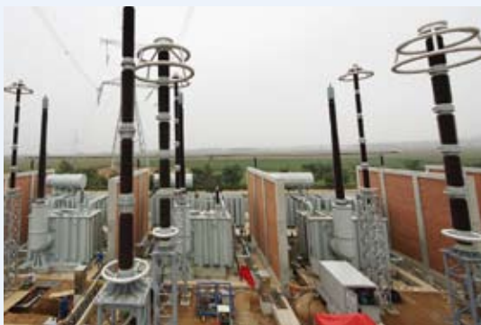
1000 kV UHV shunt reactor installed at the Jindongnan Substation, UHV AC Experimental and Demonstration Project
