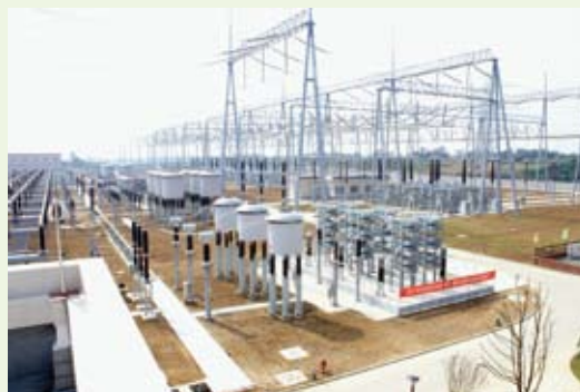
The world's first double-bridge grounding capacitor in the UHV AC pilot project
