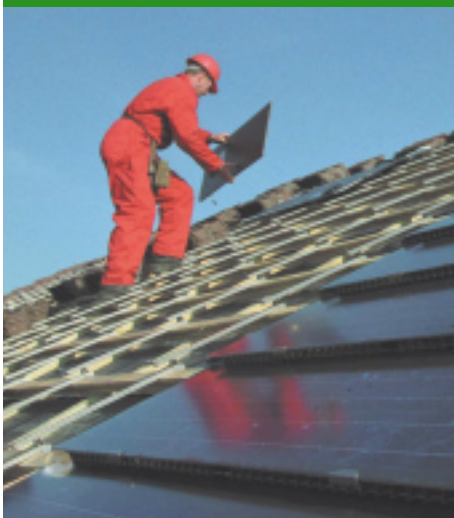
ROOFING | Installing photovoltaic systems
