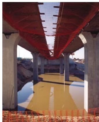
Installation of collective protection on highway overpasses (left)
