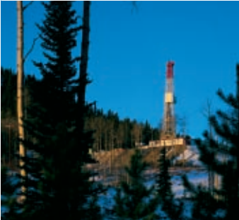
The Wildcat Hills natural gas plant in Alberta.
