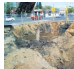
A soil excavation and back filling project in rural Saskatchewan.
