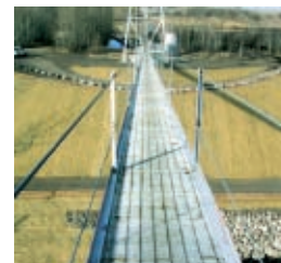
In the spring of 2004, Petro-Canada reclaimed a contaminated stretch of bank along the Bow River around the Wildcat Hills gas plant. Due to the steepness of the riverbank, safety was a major concern. The five-week operation included participation by government agencies and independent contractors.
