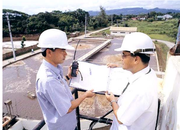
Environment Management Department staff in CADP's Wastewater Treatment Plant.
