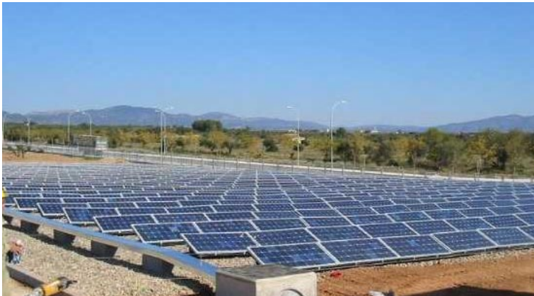
The Distribution Centre in Valls, Spain, has started to use a photovoltaic (solar cell) installation which converts sunlight into electricity. The installation is 2,700 square metres in size and has a capacity of 100 kW.
